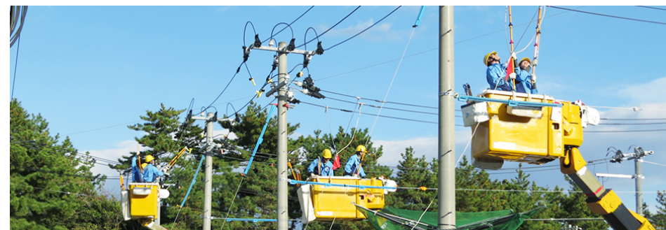
Training on pole construction using drilling and pole construction vehicles
