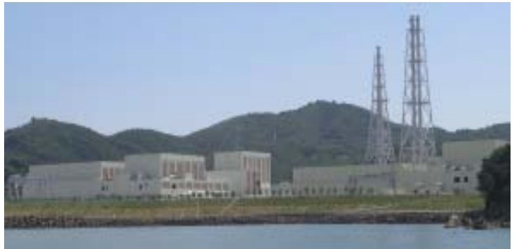
Onagawa Nuclear Power Station
