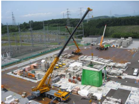
Installing 500kV equipment at Iwate Substation
