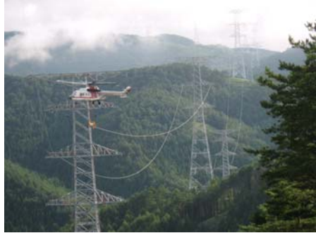
Kitakami trunk lines: Nylon ropes are stretched by helicopter
