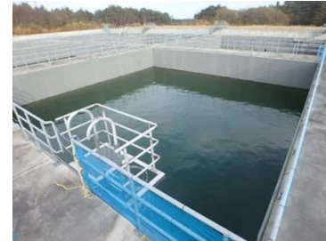
Higashidori Nuclear Power Station - Freshwater tank
