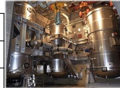
Onagawa Nuclear Power Station Reactor containment vessel filter vent system
