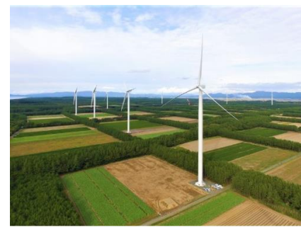
【Windfarm Tsugaru】 Output 121,600kW (Operation Started : Apr.2020)
