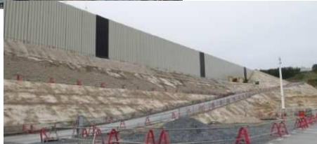
Work for raising the level of the tide embankment
