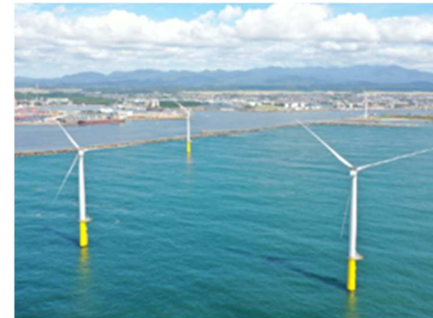
【Akita and Noshiro Port Offshore Wind】 Output 138,600kW (Operation Started : Jan.2023)
