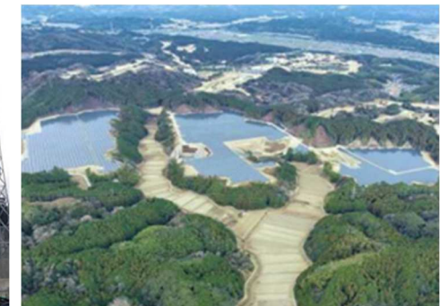
【Power Plant Tsuhaze】 Output 35,000kW (Operation Started : Feb. 2023)
