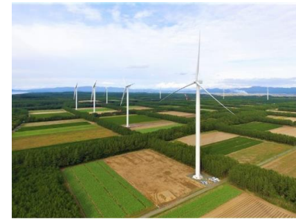
【Windfarm Tsugaru】 Output 121,600kW (Operation Started : Apr.2020)
