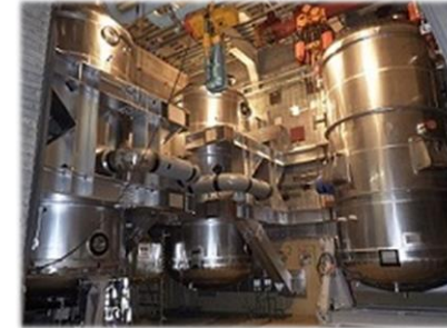
Onagawa Nuclear Power Station
