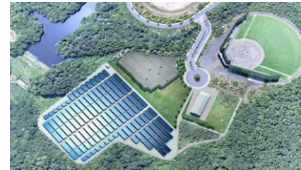
Completed image of “77 Solar Park Tomiya”
