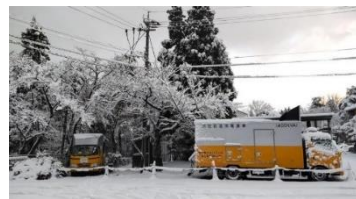
Emergency power transmission by high-voltage generator truck
