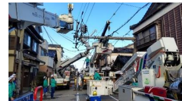
Repair of broken poles
