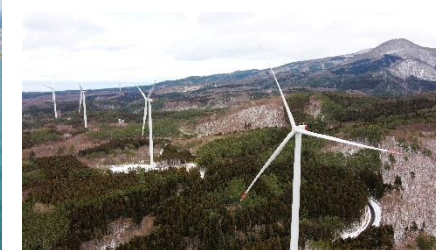
【Green Power Fukaura】 Output 73,600kW (Operation Started : Feb.2024)
