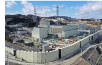
Sea wall 29m above sea level of Onagawa Nuclear Power Station
