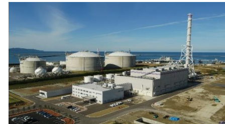
Whole View of the Joetsu Thermal Power Station
