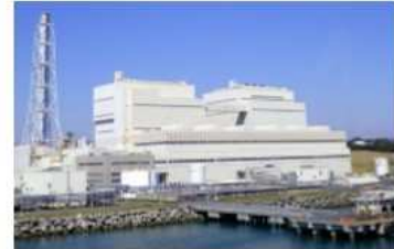
Haramachi Thermal Power Station
