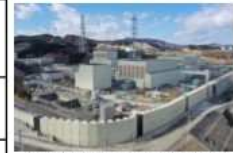
Sea wall 29m above sea level of Onagawa Nuclear Power Station
