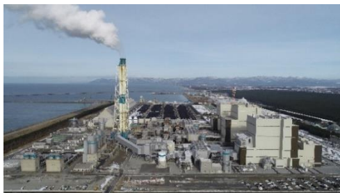
Noshiro Thermal Power Unit 3
