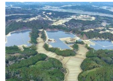
【Power Plant Tshuaze】 Output 35,000kW (Operation Date:Feb.1 2023) First participation in a renewable energy project outside of Tohoku and Niigata prefectures
