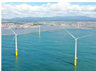
【Akita and Noshiro Port Offshore Wind】 Output 138,600kW (Operation Date:Jan.31 2023) Japan's first commercial large-scale offshore wind power project
