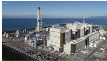
Study and verification of mixed burning of black pellets at Noshiro Thermal Power Station
