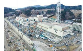
Onagawa Nuclear Power Station
