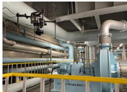
Equipment Inspection with Drone Technology
