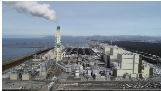
Noshiro Thermal Power Unit 3
