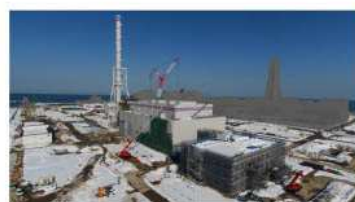
Joetsu Thermal Power Unit 1 under construction
