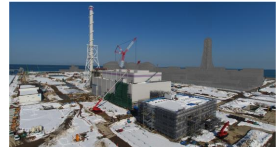
Joetsu Thermal Power Unit 1 under construction
