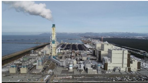
Noshiro Thermal Power Unit 3
