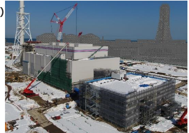
Joetsu Thermal Power Unit 1 under construction (As of January 2021)
