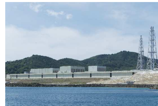
Onagawa Nuclear Power Station, where construction for safety measures is under way
