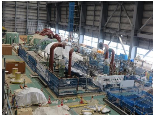
Generator and Turbine Assembly Status in Turbine Building
