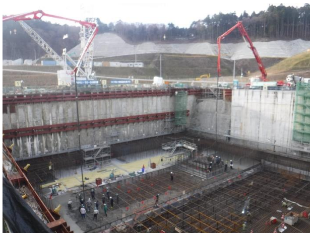
Concrete casting work of the building for emergency measures
