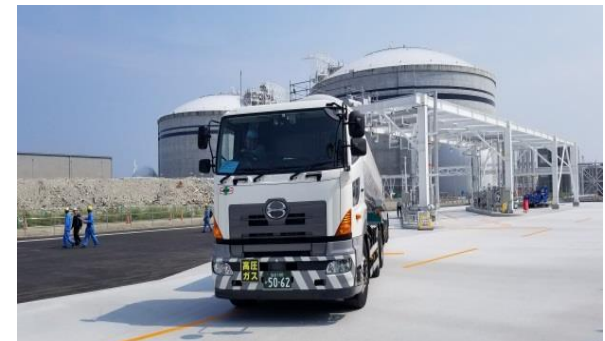
LNG Shipping Facilities of Shin-Sendai Thermal Power Station
