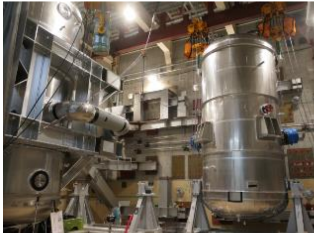
Filter vent installed in August 2018
