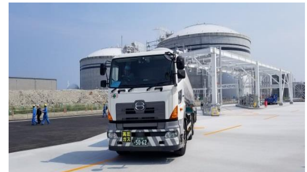
LNG Shipping Facilities of Shin-Sendai Thermal Power Station
