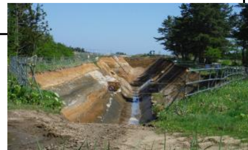
Trenching survey (Image)
