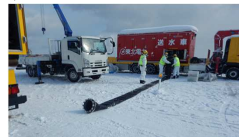
Drills in securing cooling functions with a substitute emergency cooling seawater pump (Higashidori)
