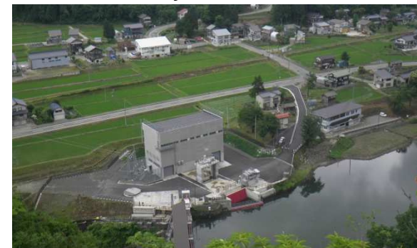
【Daini Yabukami Hydroelectric Power Station】
