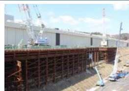
Upgrading seawall (Onagawa)
