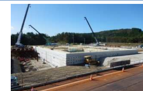
Construction of fresh water tanks (Higashidori)
