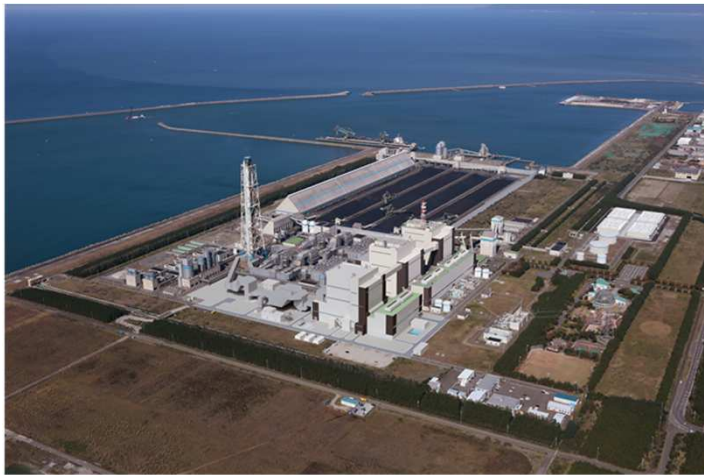
Expansion of Noshiro Thermal Power Station
