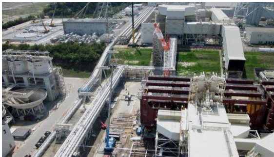
Restoration of the electric precipitator at Unit 1
