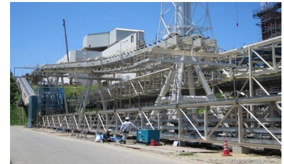
Restoration of the coal conveyer
