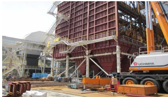
Restoration of the electric precipitator at Unit 2
