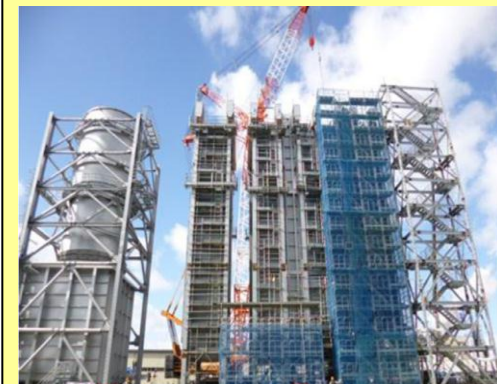
Hachinohe Thermal No.5 Upgrade to combined-cycle system
