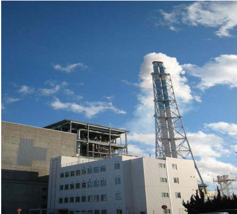
Shin-Sendai station unit No.1 (Dec.2011)
