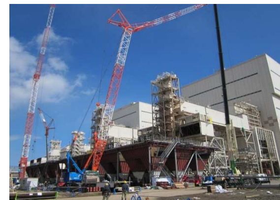
Restoration of Electric precipitator Unit No.1
