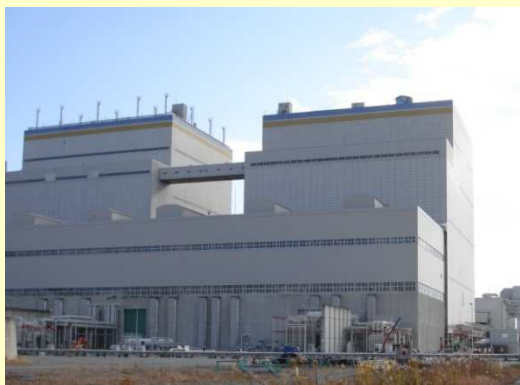
Boiler turbine building
