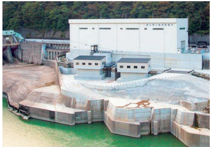
Toyomi Hydroelectric Power Station(Aga, Niigata)
