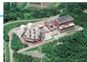
Yanaizu-Nishiyama Geothermal Power Station (Yanaizu, Fukushima)
