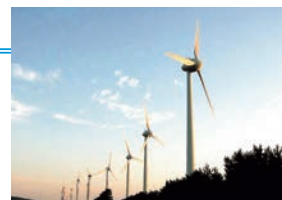
Noshiro Wind Power Station (Tohoku Natural Energy Development, Noshiro, Akita)
