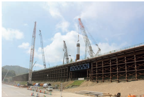
Work to raise the seawall height (Onagawa)
