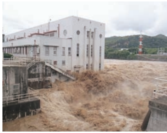
Flooding after heavy rains
