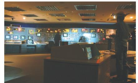
Simulation of operation on the assumption of loss of all AC power supplies
