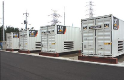
Large-scale power supply units installed at Higashidori Nuclear Power Station to ensure power supplies in an emergency
