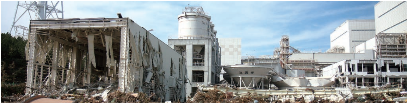
Haramachi Thermal Power Station(March, 2011)
