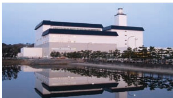
Sendai Thermal Power Station No.4
