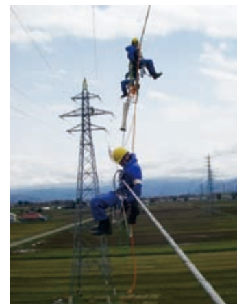
Inspection of Cables
