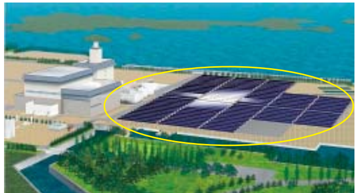
Sendai Thermal Power Station Site (rendering) Output: Approx. 2,000 kW, Reduction of CO 2 emission: Approx. 1,000 tons annually (estimate)
