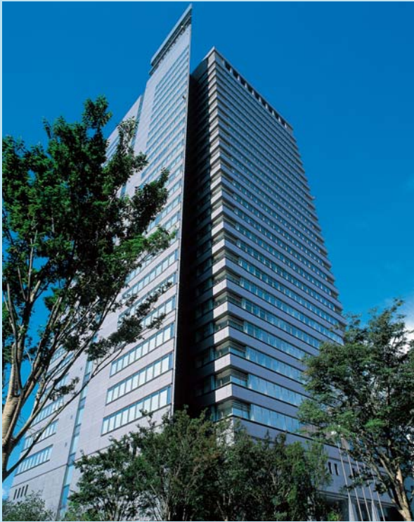
Head Office (Sendai City, Miyagi Prefecture, Japan)
