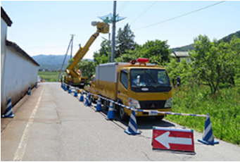
Placing safety barriers around the work area
