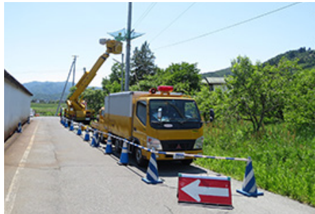
Placing safety barriers around the work area
