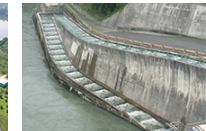
Fish ladder at dam
