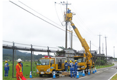
Positioning traffic guide personnel
