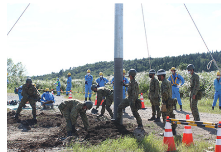
Recovery work drills assuming blocked roadways [Ground Self-Defense Force]
