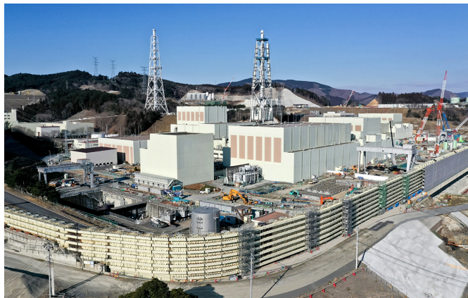
Progress on seawall construction (Onagawa Nuclear Power Station)
