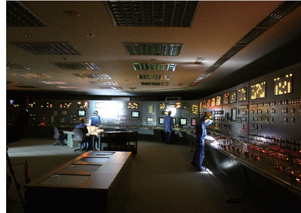
Operational training using a simulator, assuming an accident in which all AC sources are rendered unusable (Nuclear Power Operation and Maintenance Training Center)
