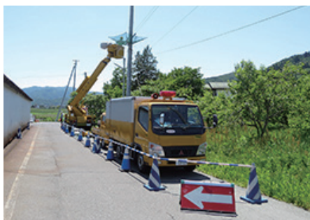
Placing safety barriers around the work area
