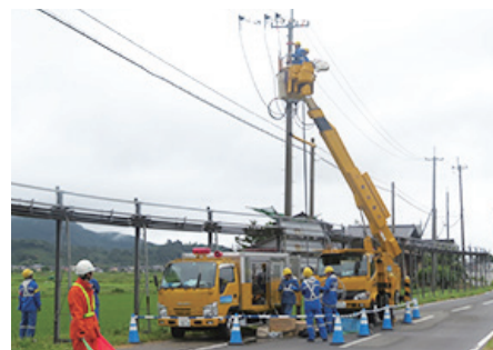
Positioning traffic guide personnel
