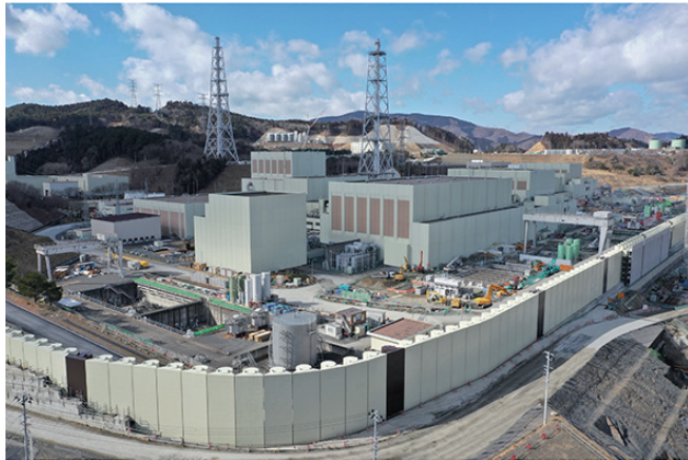
Progress on seawall construction (Onagawa Nuclear Power Station)
