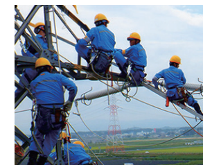
Training on installing cable fixtures in transmission engineering section
