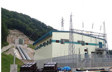
New Tamagawa No.2 hydroelectric power station (completed in November 2022)
