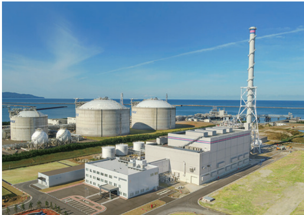
Unit No. 1 at the Joetsu Thermal Power Station began operating commercially in December 2022.
