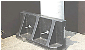
Plastic deadman (buried in the ground to prevent power pole collapse)
