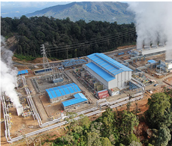
Rantau Dedap Geothermal Power Plant (Indonesia)
