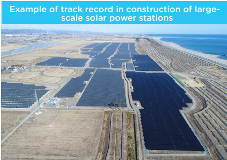
Watari Solar Power Station • Comprehensive construction contract • 79,458 kW • 22 kV on-site power lines • 66 kV/22 kV transformer facility
