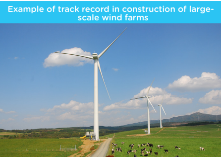
Rokkasho Futamata Wind Farm • Comprehensive construction contract • 1,500 kW turbines × 34 • 22 kV power line (20 km) • 154 kV power line (1.2 km) • 154 kV/22 kV transformer facility
