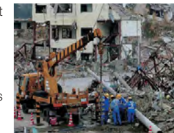
Utility pole erection work immediately after the earthquake
