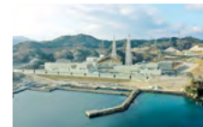
Onagawa Nuclear Power Plant, where safety construction is underway
