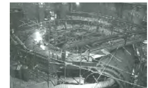
Scene from the construction of Numazawa Power Plant No. 2
