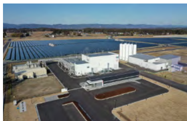
Aerial photo of the Name Fukushima Hydrogen Energy Research Field (FH2R) project
