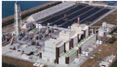
Unit No. 3 at the Noshiro Thermal Power Plant
