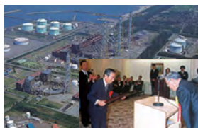
Higashi Niigata Thermal Power Station series 4-1 achieved world-class thermal efficiency levels exceeding 55%.
