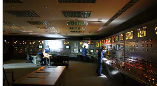
Operational training using a simulator, assuming an accident in which all AC sources are rendered unusable (Nuclear Power Operation and Maintenance Training Center)
