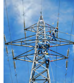
Transmission line grounding installation and removal training in power transmission section
