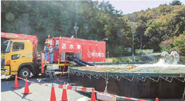
A drill on use of a large-capacity pump truck to pump water to nuclear reactors and spent-fuel pools in an emergency (Onagawa Nuclear Power Plant)
