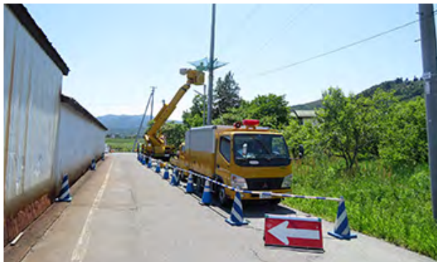
Placing safety barriers around the work area
