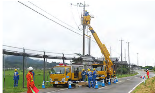
Positioning traffic guide personnel
