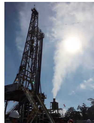
Lantau Dedap Geothermal Power Plant under construction (Republic of Indonesia)
