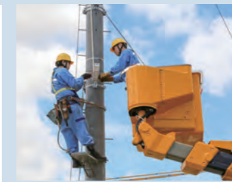
Donated street light installed in Namie Town
