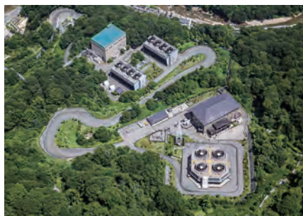
Kakkonda Geothermal Power Station
