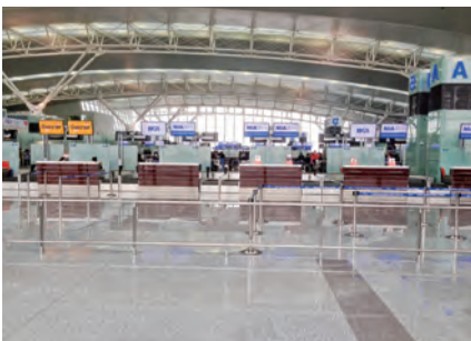
Noi Bai International Airport (Vietnam) (Installation of electric equipment)
