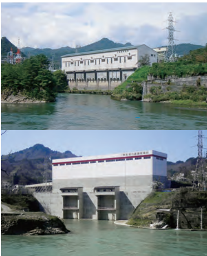
Upgrade of Kanose Hydroelectric Station (Above: Before upgrade, Below: After upgrade)
