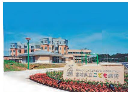
Miyagi Children's Hospital (ESCO project)
