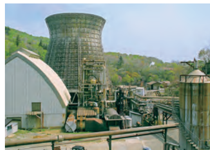
Matsukawa Geothermal Power Station
