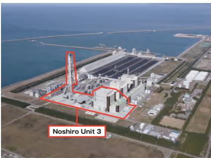
Construction Image of Noshiro Unit 3
