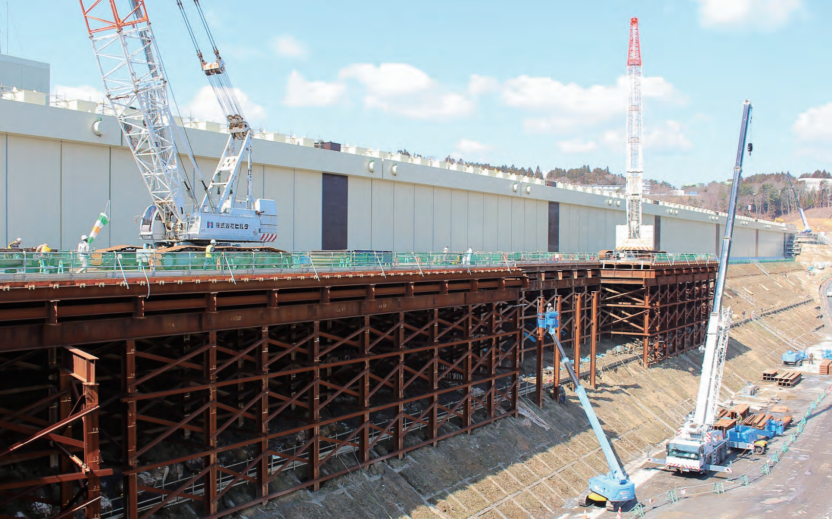
Upgrading the seawall at Onagawa (March 2017 photo)
