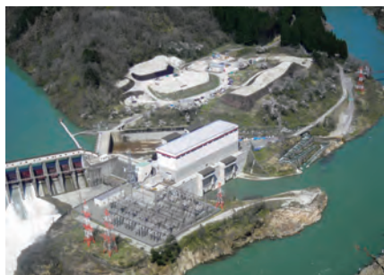
Kanose Dam (constructed in 1928) and Kanose Power Station under upgrade (to be completed in 2017).
