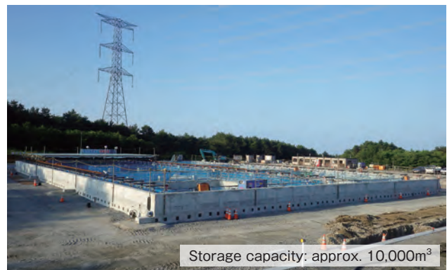
Construction of fresh water tank at Higashidori (May 2017 photo)
