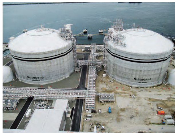
LNG tanks on the premises of Shin-Sendai Thermal Power Station
