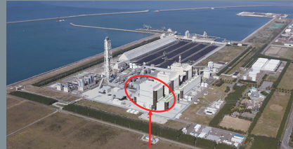
Noshiro Thermal Power Unit 3 Construction Image
