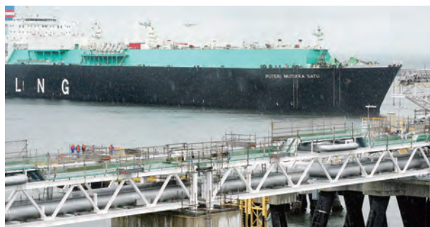
An LNG tanker approaching Shin-Sendai Thermal Power Station
