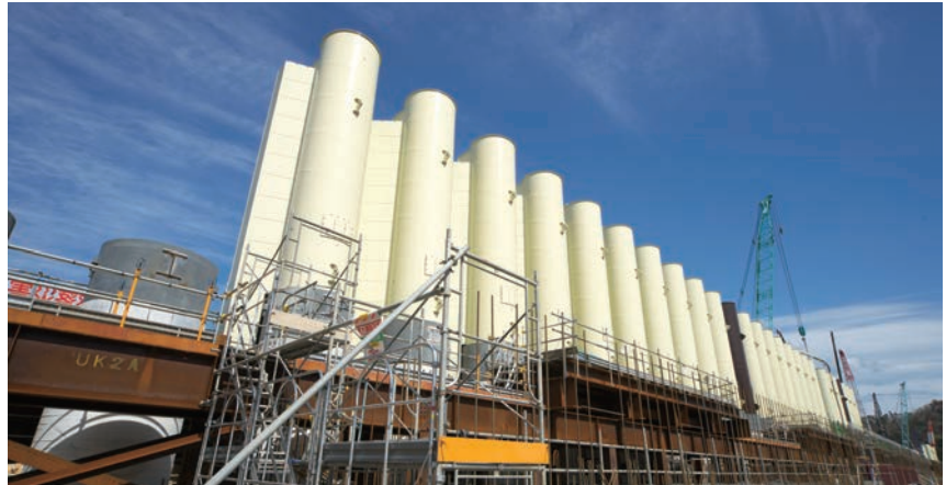
Safety Seawall at Onagawa
