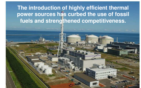
Joetsu Thermal Power Station Unit 1
