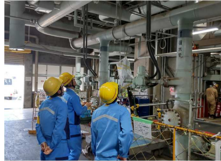
Conducting safety patrols
