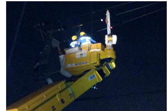
Power restoration support after an outage caused by Typhoon No. 15 (September 2019)
