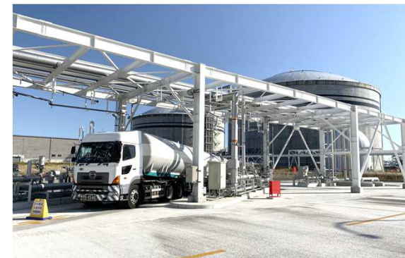
LNG shipping facility at Shinsendai Thermal Power Station
