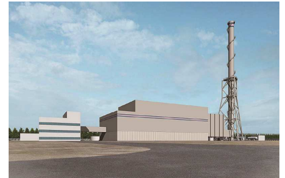
Joetsu Thermal Power Unit 1, which aims for the world’s highest level of thermal efficiency of 63% or more (Commercial operation planned to start in June 2023)
