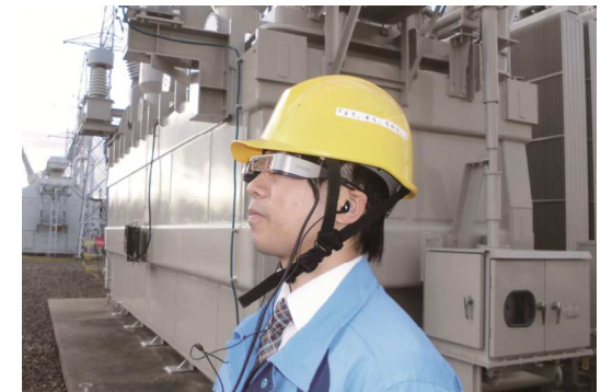
Operation of a smart glass system to improve the quality and efficiency of substation operation and maintenance
