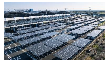
On-site PPA Case: Carport-type Solar Power Station at Sendai Airport (Photo: Sendai Airport Re-Energy Power Generation LLC)
